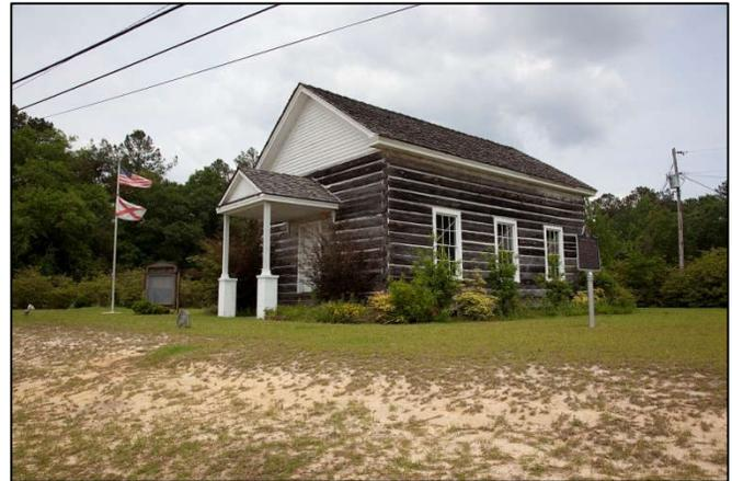
The squared-log building features square notched corners and a wood shingle roof. It is a single pen log structure which measures 36 feet by 26 feet and rests on 10 brick piers 18 inches in height.
